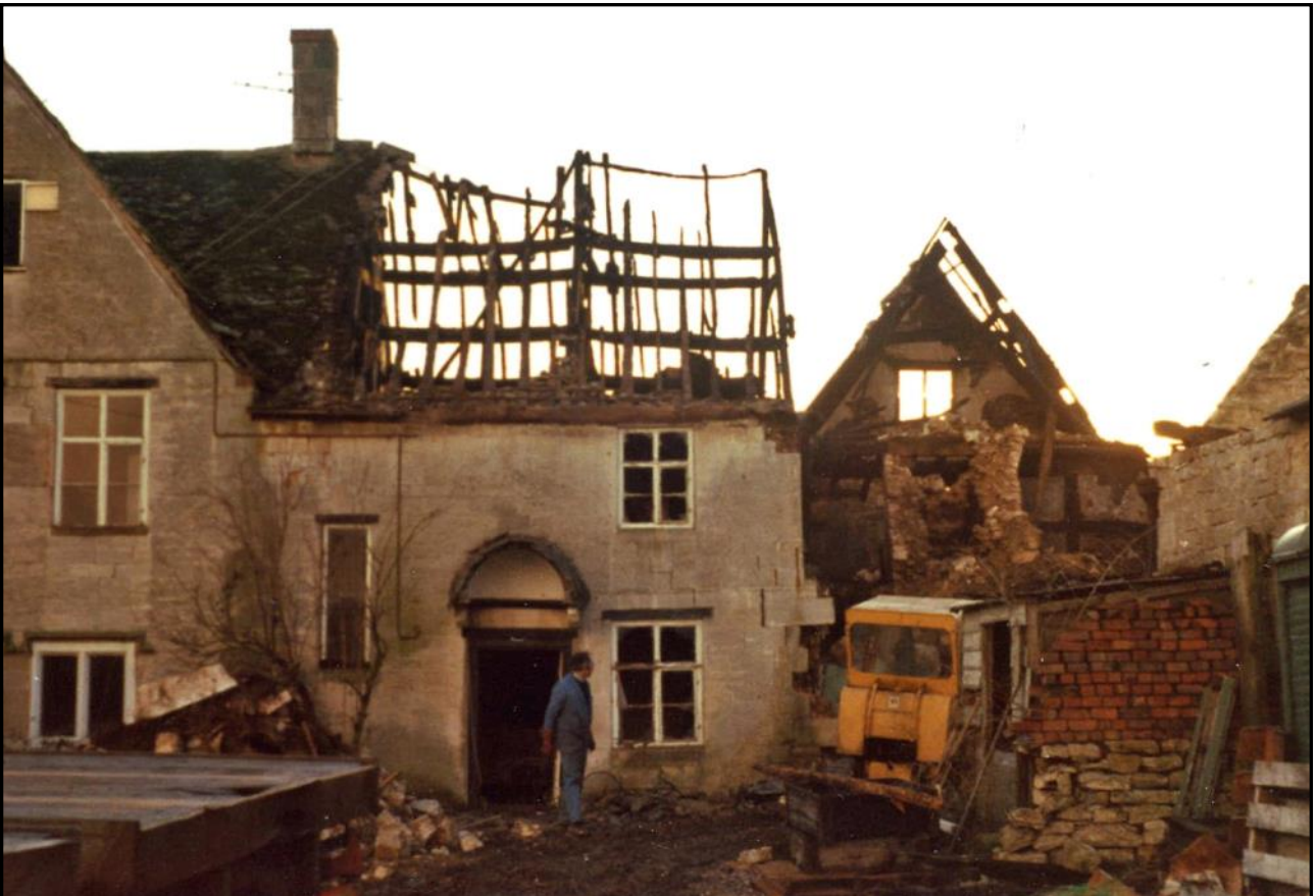
Oldends Hall from the north-east after the fire, showing the damaged roof timbers of the medieval hall and extended service block.
