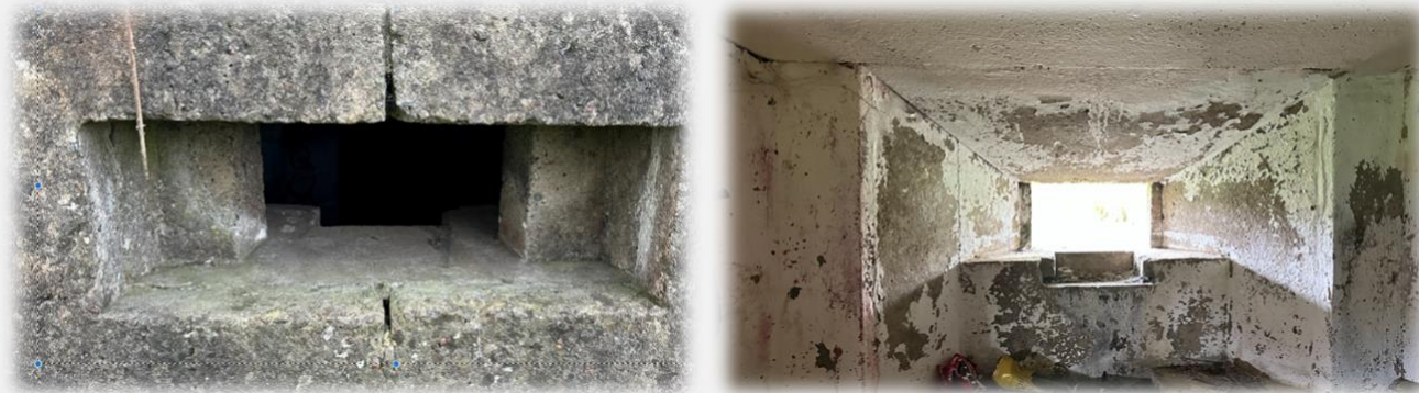
Figure 11 and Figure 12: External and internal views of an embrasure
