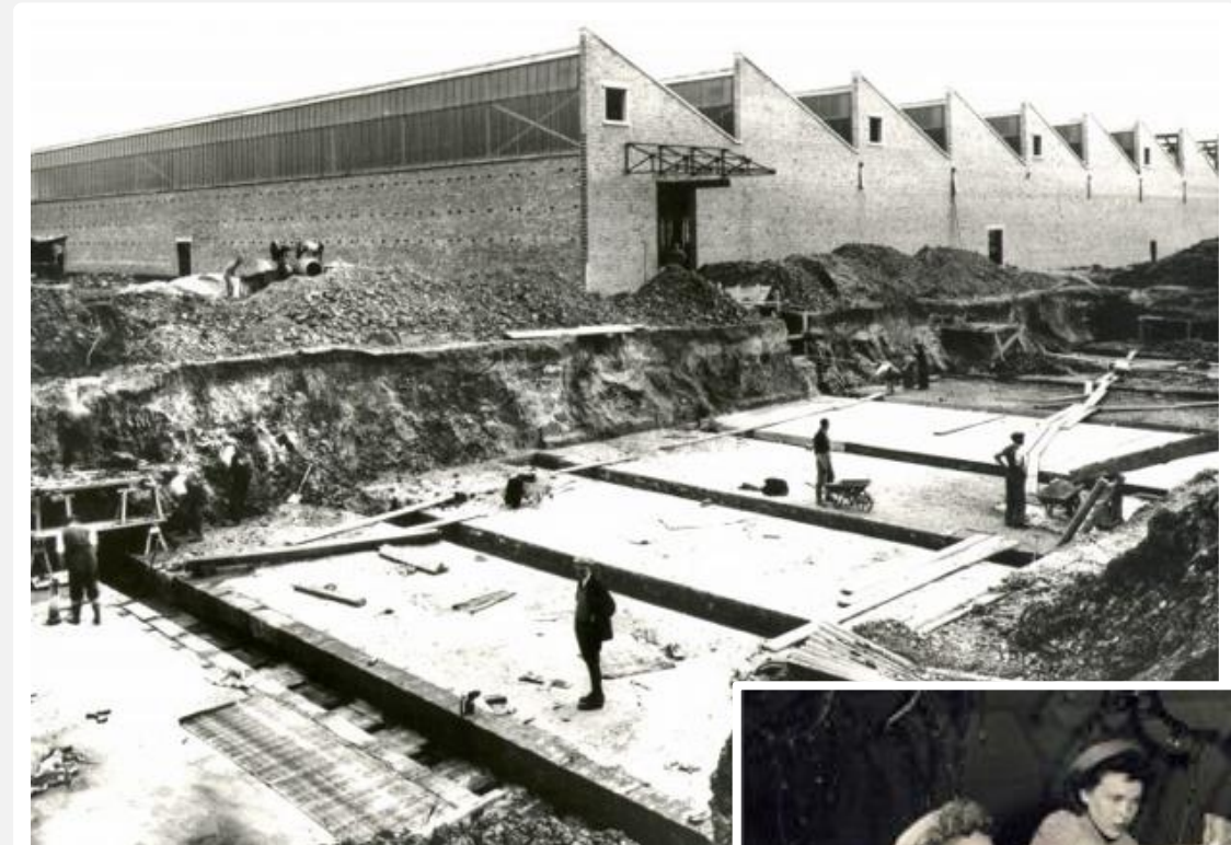
Figure 21: Construction of the Hoffman shadow factory 1939-1940 © Hoffmann Bearings
