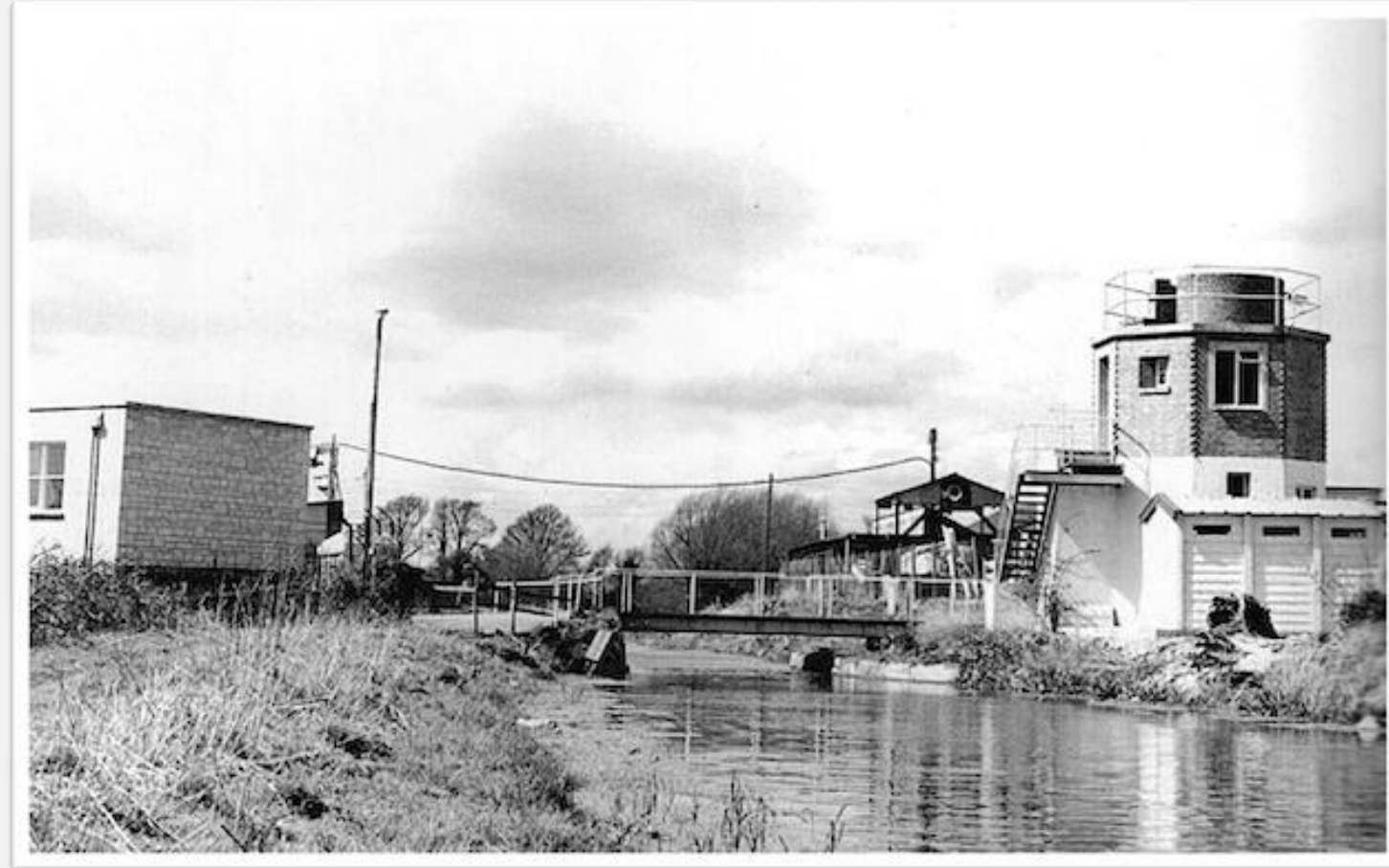
Figure 14: 1970s photo showing the swing bridge and pillbox © M. Handford
