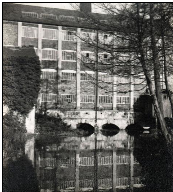
The rear of Stanley Mill showing the engineering workshop with Club and Billiard Room on top two floors.
