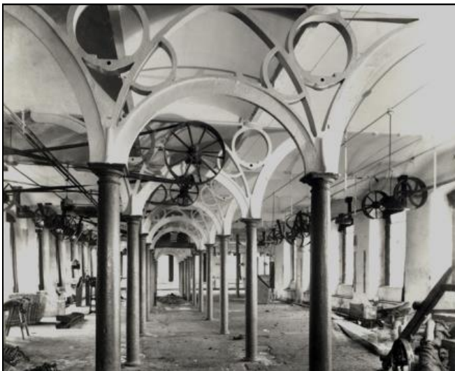
The interior of Stanley Mill ©Peckham's Photos
