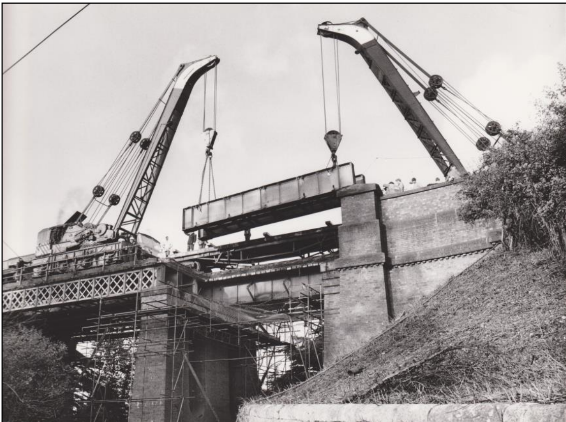
Figure 6. Two rail-mounted cranes removing part of the 1884 deck in 1971.
