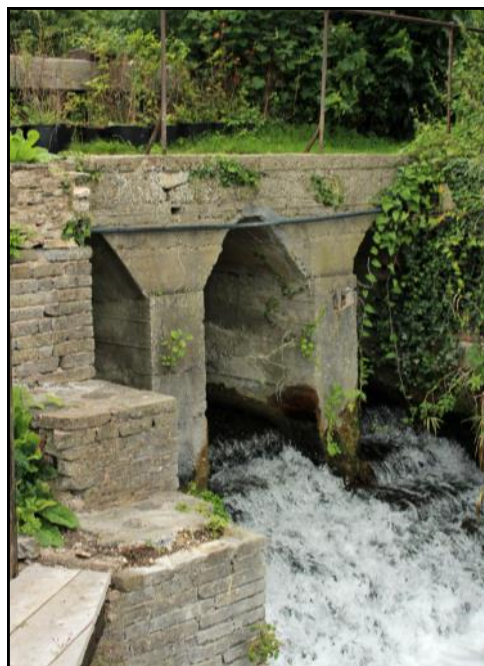
Weir at Churchend Mill looking north east, August 2017.
