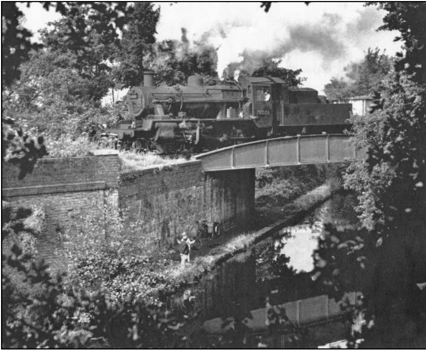
Steam locomotive crossing Skew Bridge on 23rd August 1965. The brick retaining wall and the towpath on the southern bank are clearly visible.
