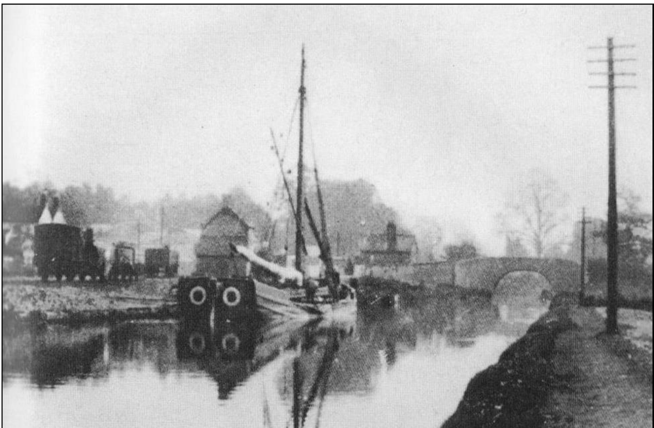
Stonehouse Wharf c.1900. Note the railway wagons on the siding to the left of the boats.
