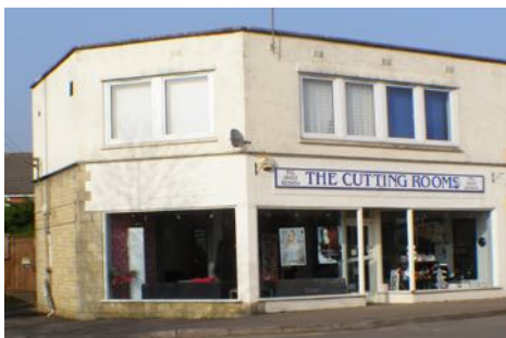
Formerly the Rodney Lewis Electrical Goods Shop.
