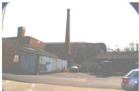
On the top floor of this Marling and Evans mill building, was, I think, the room where the Rock'n'Roll Dances were held
