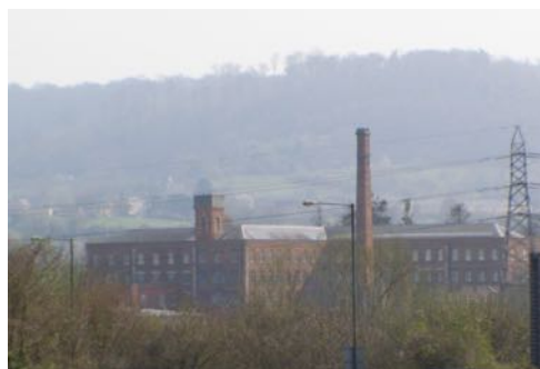
The Marling and Evans mill building, Ryeford/Kings Stanley
