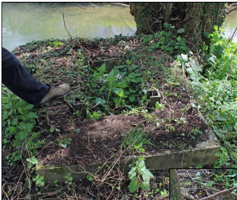
Figure 9: Probable inlet for water from the Frome at the eastern (Stanley Mill) end of the plantation. Pair of iron channel pieces still in place which would have carried a stop board some 2 feet wide. Some form of pump was probably necessary to lift the water from the Frome at this location.
