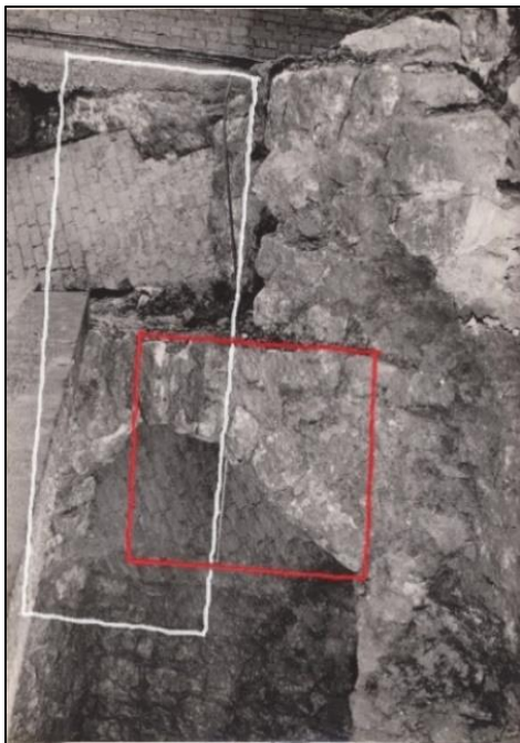
Photo 2: detail of photo 1, area edged white, from along the plank, shows lower skin of brick vaulting continuing behind stone arch and resting on stone wall
