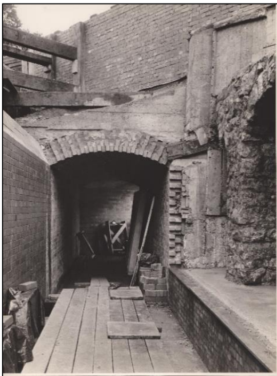
Photo 4: looking south towards the High Street, shows brick and concrete work 1957
