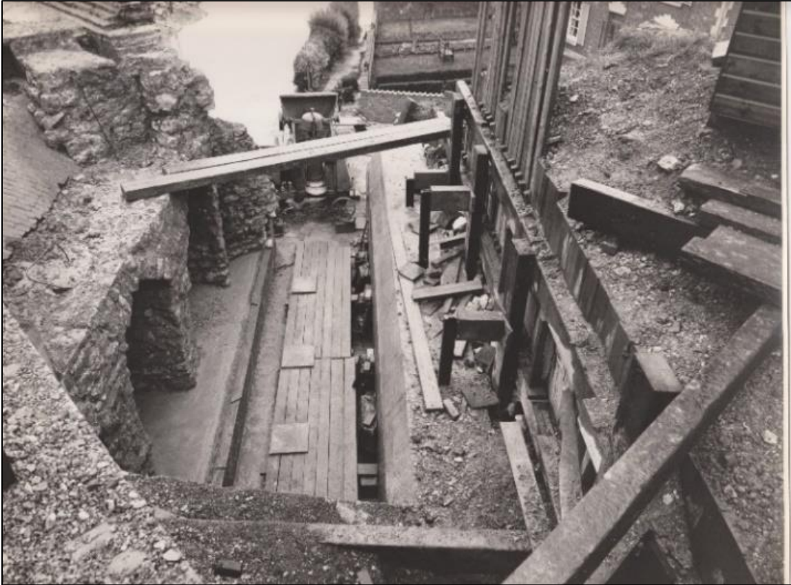
Photo 5: aerial view, looking north, shows stone arches aligned with presumed course of stream in culvert: remnants of stone added above the brick vault, metal ties used to secure it, and stump of angled stone wall across front of the embankment: 1 and 3 Gloucester Road visible on right
