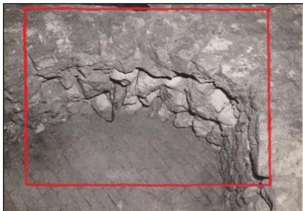
*Photo 3: detail of photo 2, area edged red, looking up under stone arch, shows roughly finished surface, and metal tie*
