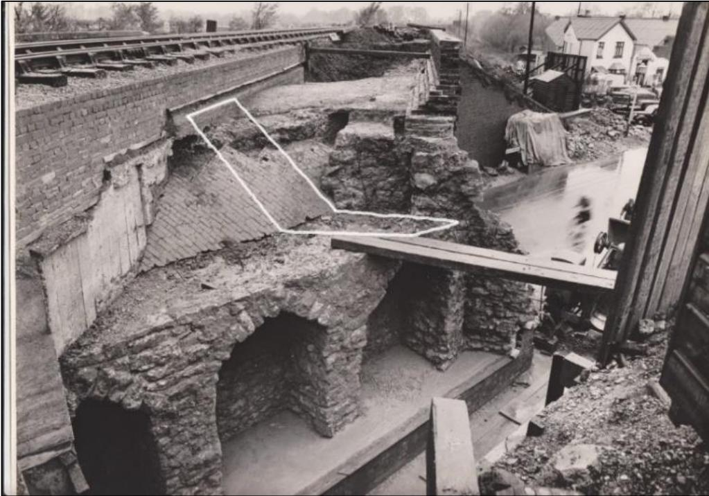
*Photo 1: looking west, shows higher skin of brick vaulting resting on the stone arches, stone wall under bridge behind arches, stub of end stone wall*
